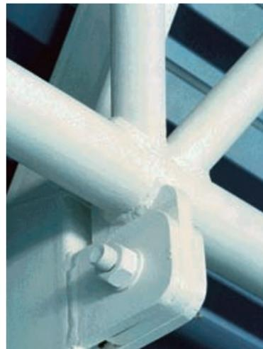
Hollow round, or square sections are most frequently chosen for their visual appearance. **Sika® Unitherm®** intumescent coatings give protection against fire without affecting the appearance of the structure. The range of **Sika® Unitherm®** decorative finishes will also enhance the appearance of the structure.
